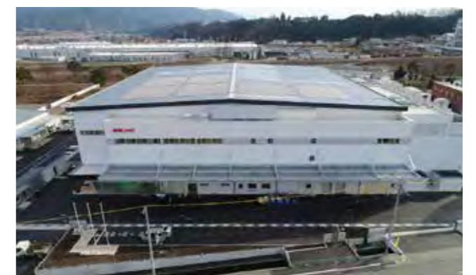
NHK Spring Miyada Plant (144kW, Start from FY2018)
